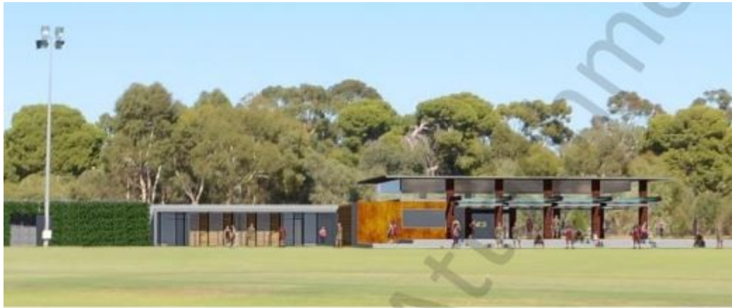
View from East (Oval & Mann Road)
