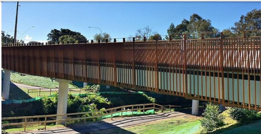
Alongside Hackney Road, a new shared-use bicycle and pedestrian bridge over the Torrens has been opened .
