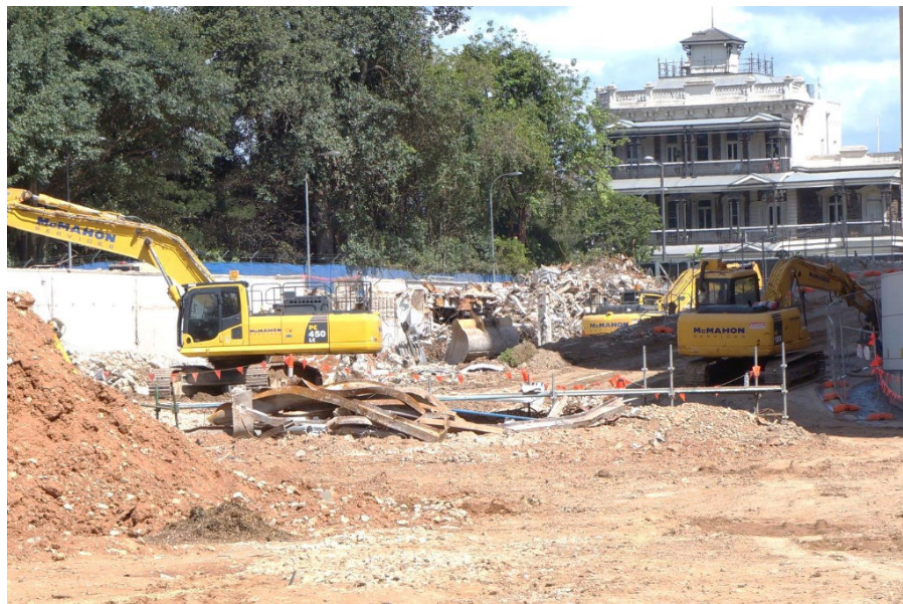
Demolition of F S Hone and East wings
