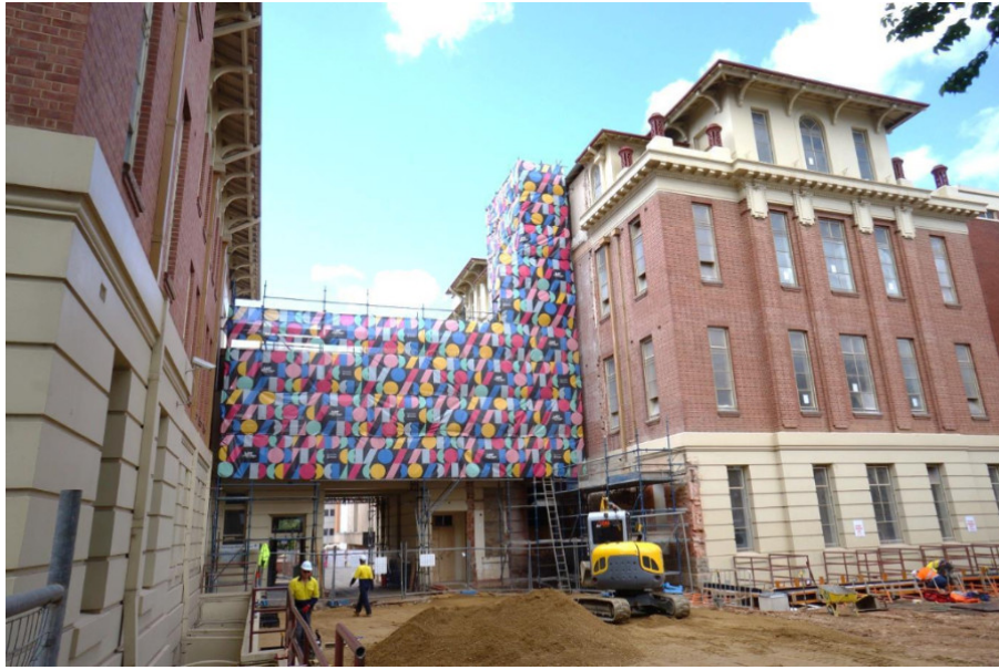
Outpatients (L) and A & C (R) buildings undergoing renovation
