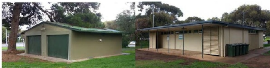
Existing Maintenance Shed
