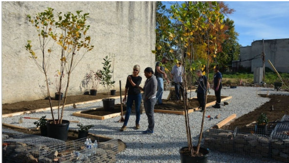
Volunteers building a "pop-up park" in Pittsburgh, Pennsylvania
