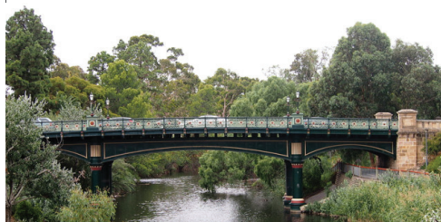
The Albert Bridge
