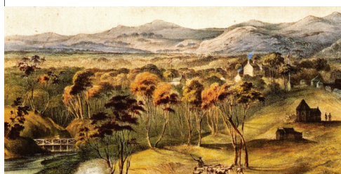
E.A. Opie: the first bridge over the Torrens.
