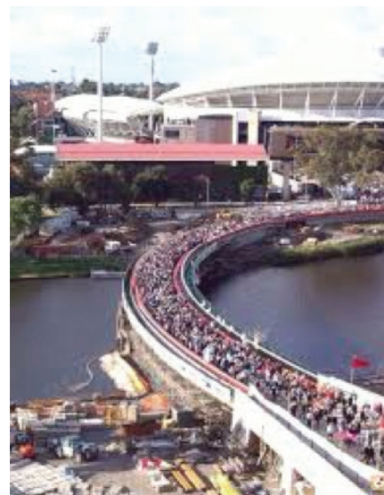
The new but as yet unnamed footbridge to Adelaide Oval
