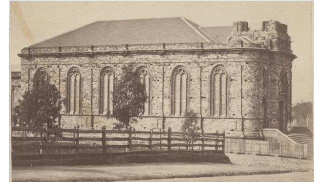
The tower was added in 1871.
