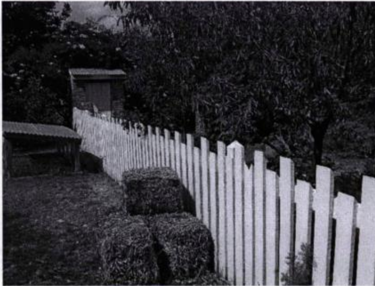
Fence and WC to rear former Magazine Keeper's Residence
